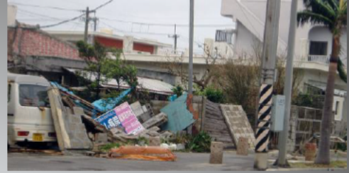
Damage caused by Typhoon Shanshan (2006) Based on the observation by Fudeyasu's research group, the isotope of water vapor in the eye of the typhoon was successfully measured for the first time in the world.
